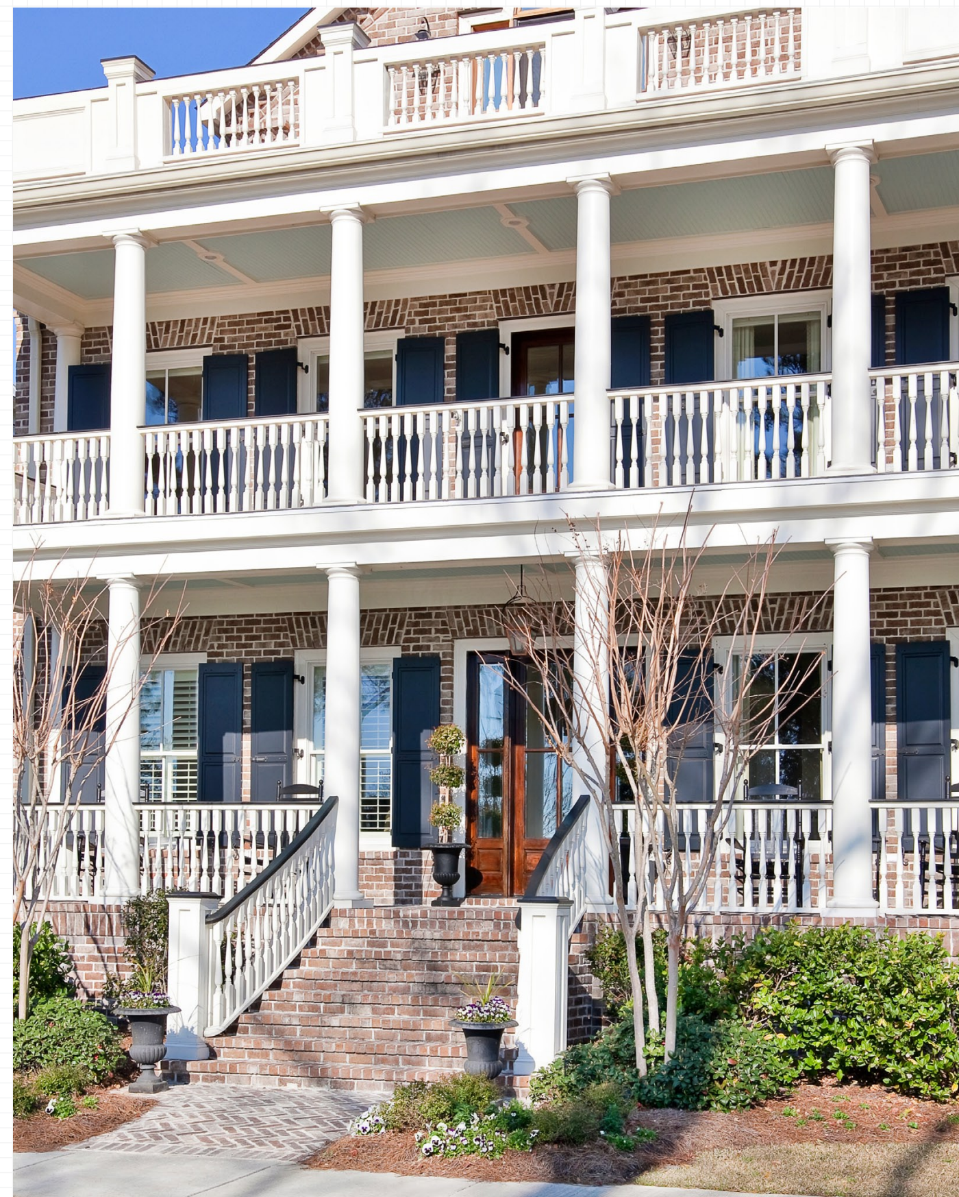
The classic Lowcountry-style façade of the home includes colonial shutters and wide balconies.
