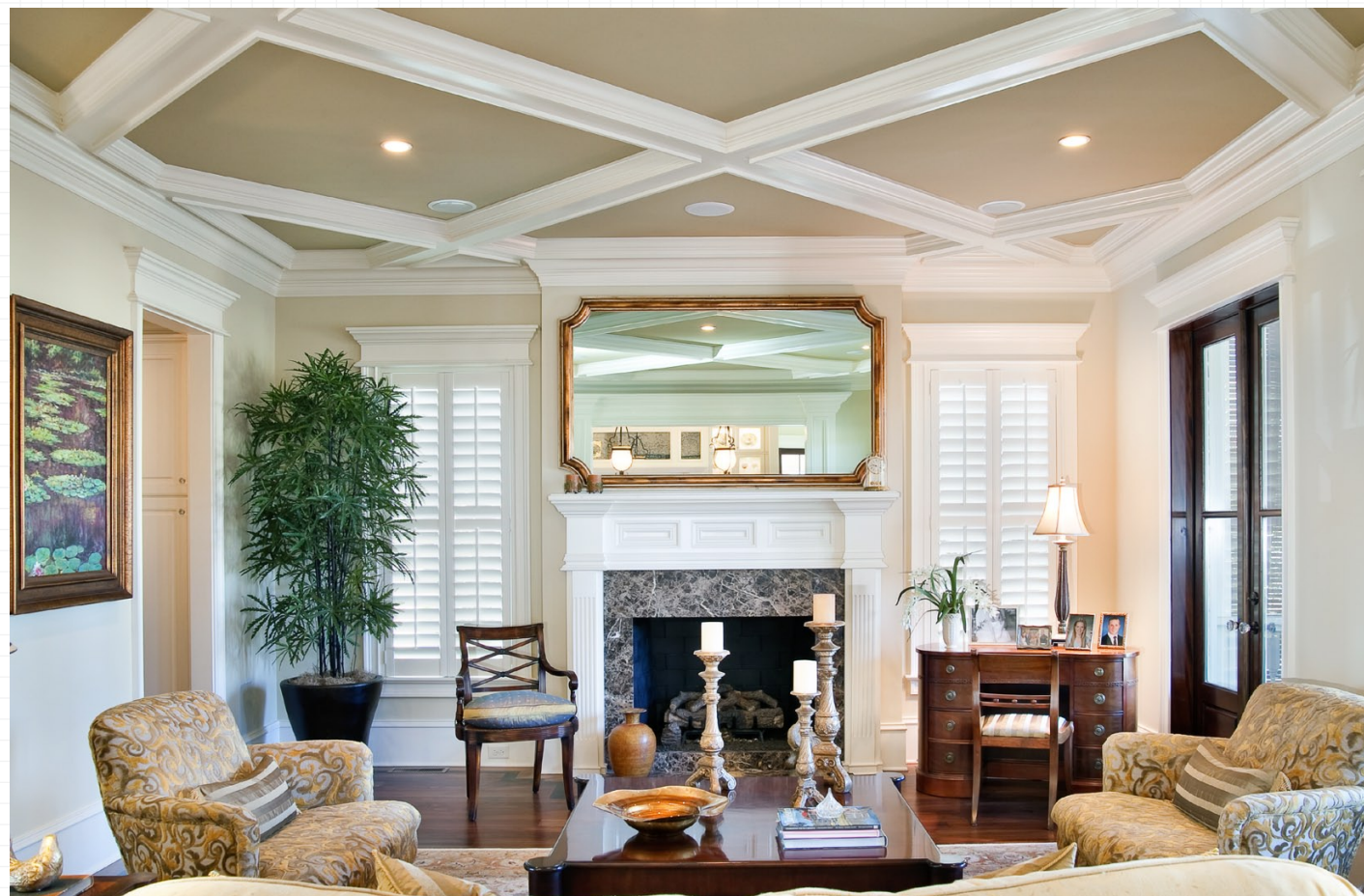
The living room of the Quinlan family's Daniel Island home is rife with architectural details such as coffered ceilings, crown moulding, and plantation shutters. A custom two-way mirror above the mantle hides the television, making it virtually invisible to the naked eye when not in use.
